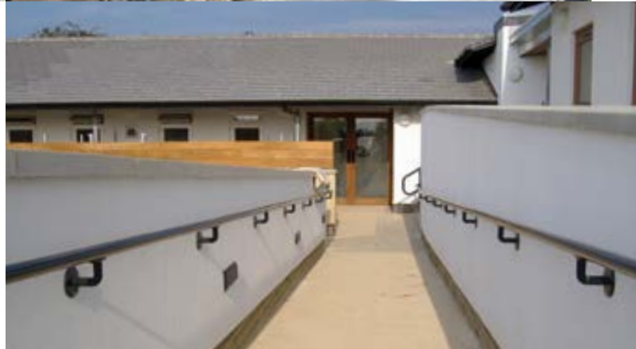
Right: ADA Compliant Railing for Access Ramps
